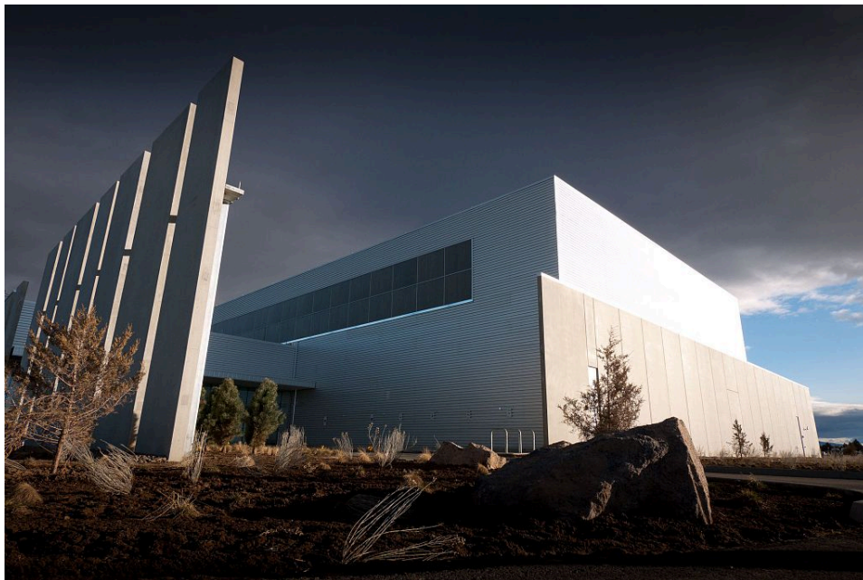
Figure 4.4: Data centers, such as this one housed in Oregon in the US, are major investments to both build and operate (Source: By Tom Raftery (Flickr) [CC-BY-SA-2.0 ( http://creativecommons.org/licenses/by-sa/2.0 )], via Wikimedia Commons).
